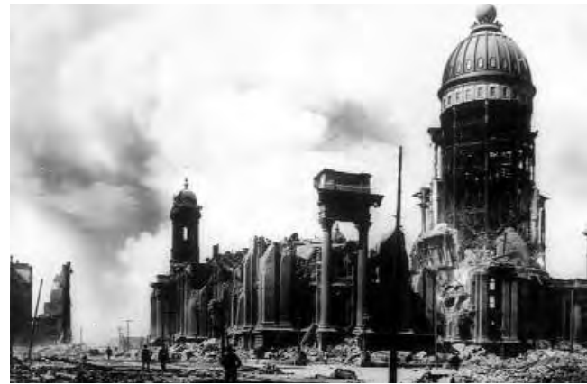
Shaken and burned. The U.S. Geological Survey described San Francisco’s City Hall as “a monument of bad design and poor materials and workmanship” (2).
