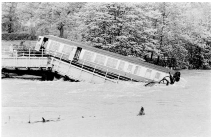
Fig. 3.1 Llandeilo train crash, October 1987: collapsed bridge
